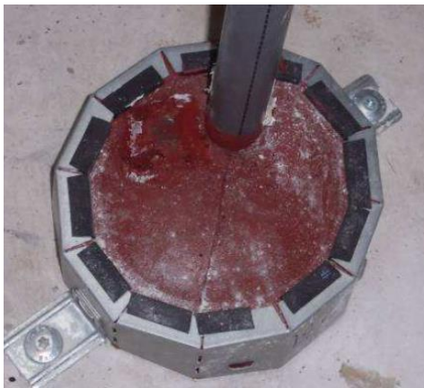
Figure 3 Optional rubber protection strip on edge of collar
