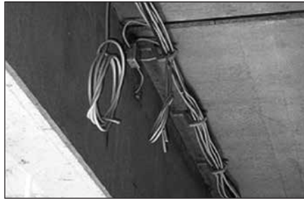
X-ECH for fastening bunched cables
